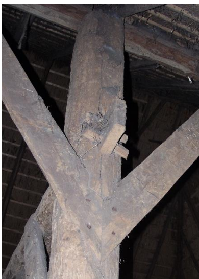
96. Verbinding ankerbalk.
